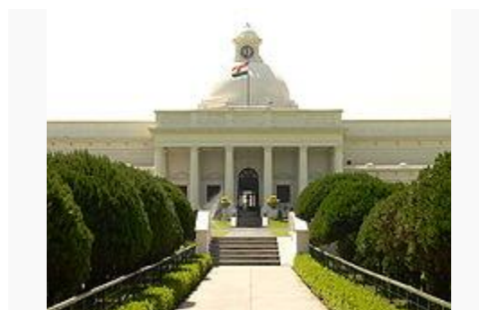
Main (Administrative) Building, IIT Roorkee
